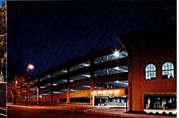
Valdosta State University Parking Structures, Valdosta, Georgia
