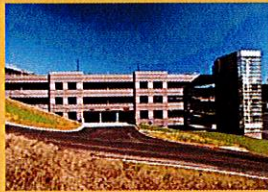
Southern Polytechnic State University Parking Structure, Marietta, GA
