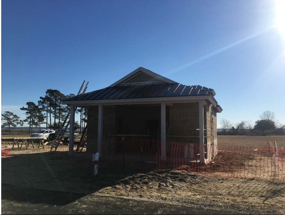
Photo No. 1 Description: Front Elevation.
