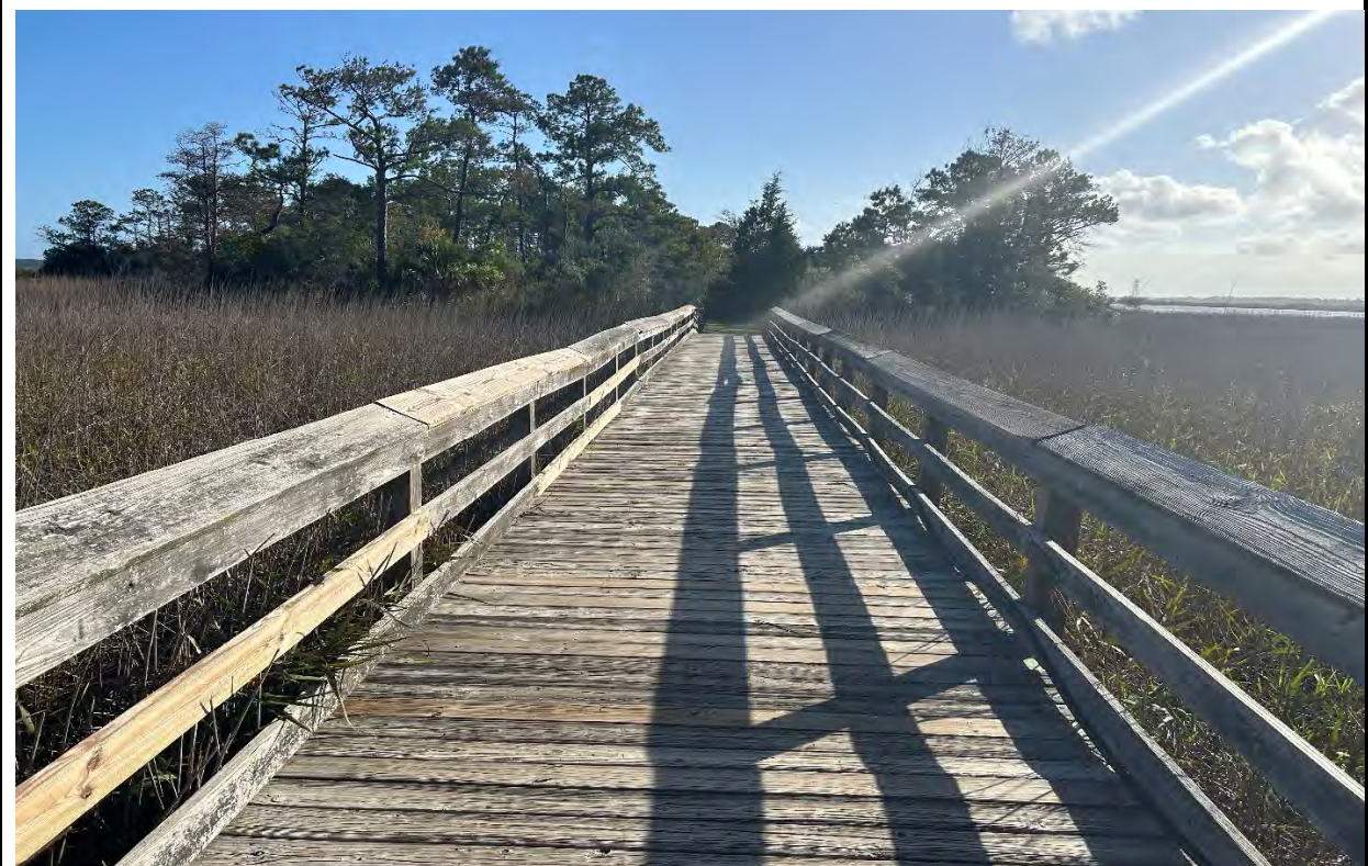
Photo No. 6 Description: Wood bridge leading to tree area
