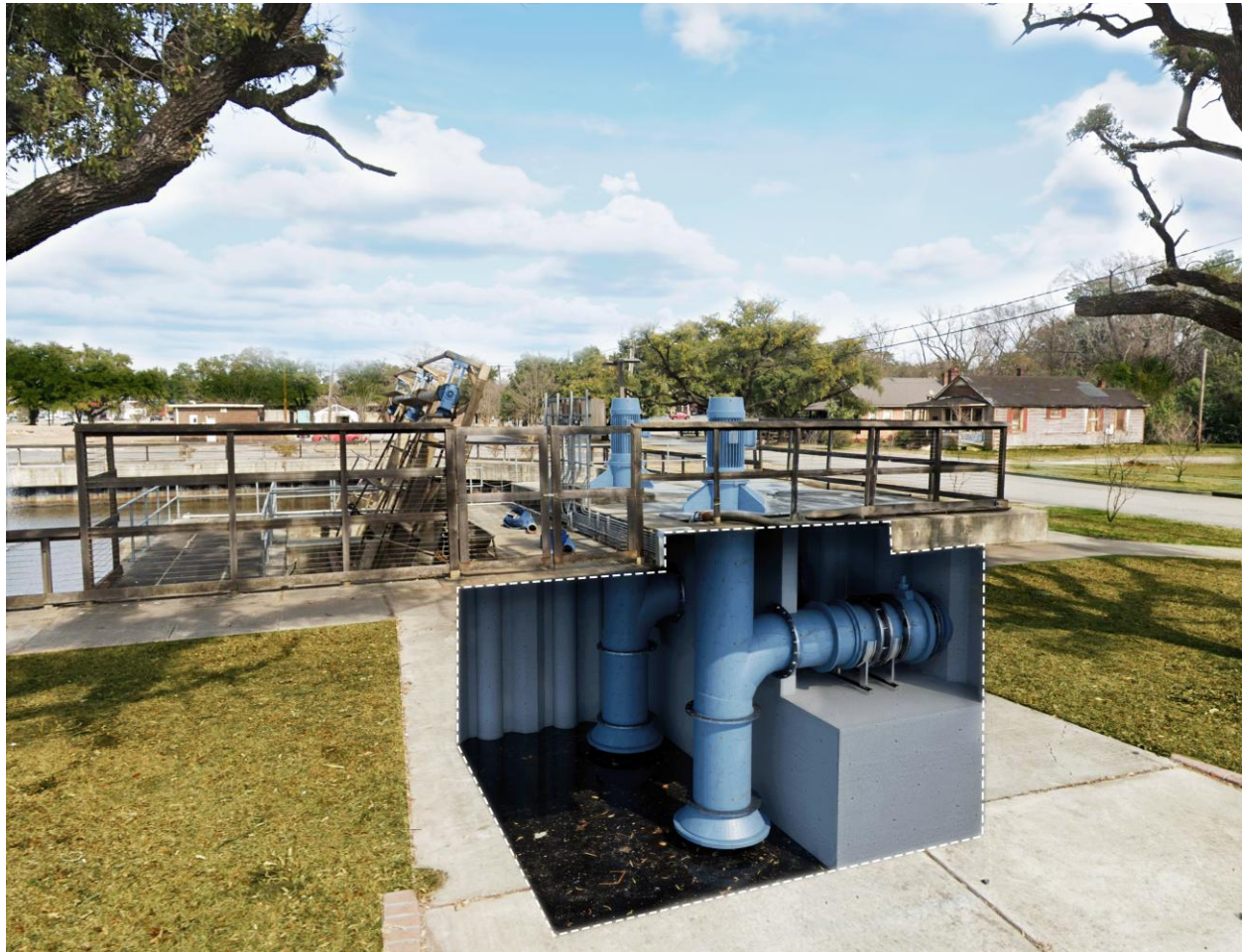
Figure 8 – Vertical Axial Flow Pump with Direct-Drive Motor Rendering
