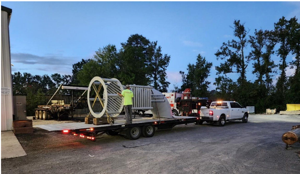
Figure 13 – Delivery of existing MWI hydraulically-driven submersible pumps
