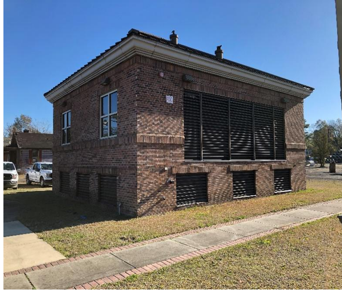
Figure 4 – Existing Motor House at 1224 Front Street
