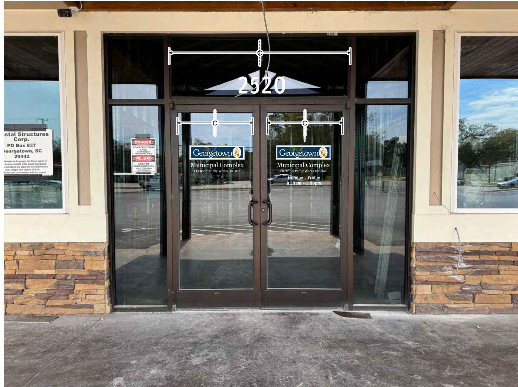
INSTALLED VINYL Photo Edit | NTS
