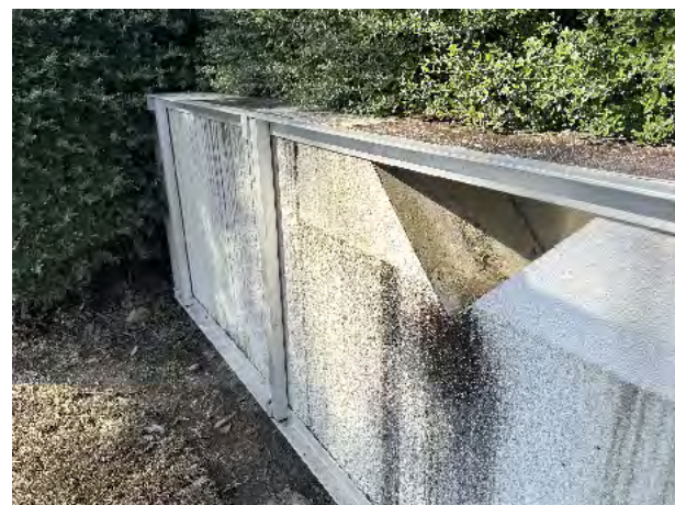
ADDITIONAL EXISTING SIGN PHOTOS For Reference Only – NTS
