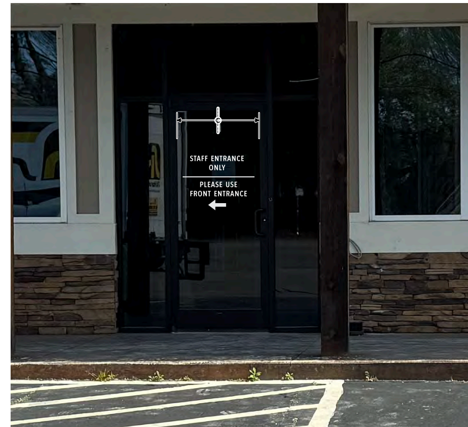
D5 INSTALLED VINYL - TYP. Photo Edit | NTS
