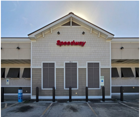
Existing Store Front
