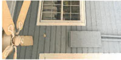
Relocate existing electrical panel
