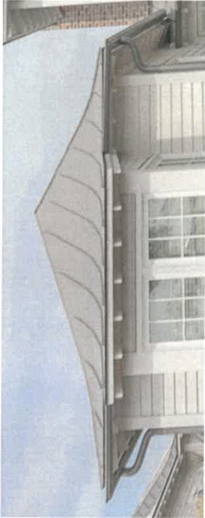
Dark hand crimped standing seam metal roof at proposed Garage
