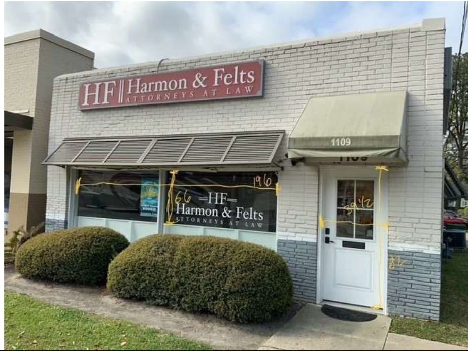
EXISTING FRONT ELEVATION IMAGE
